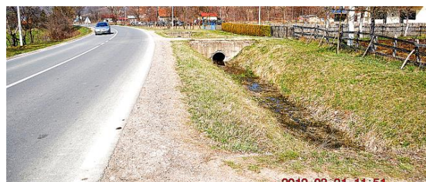
Unsafe drainage system, U-Type with headwall
