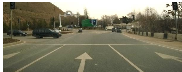
Missing channelisation in junction
