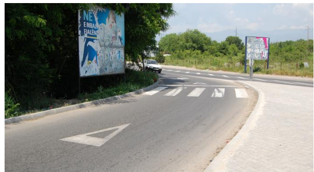
Missing of pedestrian footpath
