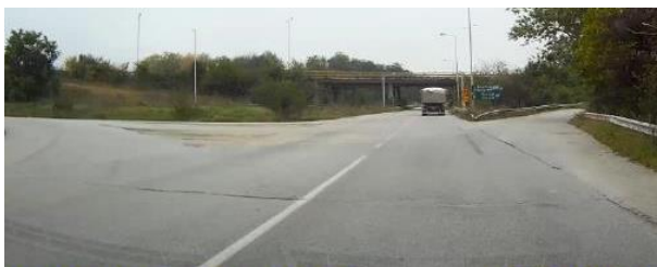
Missing channelisation in junction
