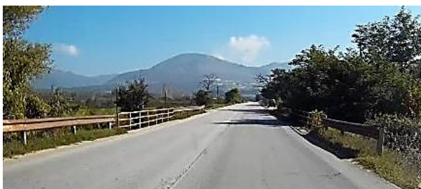
Dangerous guardrails (not a system)
