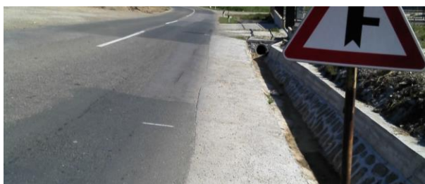
Unsafe drainage system, with headwall
