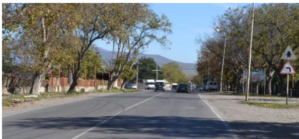
Sharp left curve + optical illusion (secondary road in curve gives perception that road is going straight)
