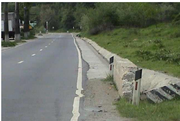
Unsafe headwall of a culvert
