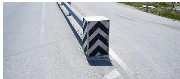
Dangerous “end treatment”- concrete block
