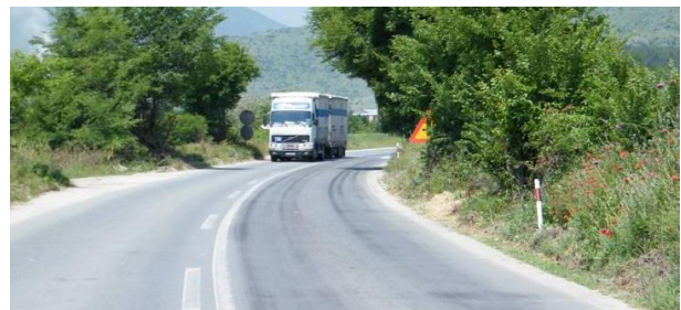
Insufficient site distance in curve
